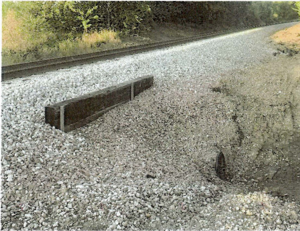
FIGURE 4: EXISTING CULVERT UNDER IAS RAILROAD, EAST OF AT-GRADE CROSSING, LOOKING EAST
