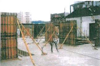
**EFCO HAND-E-FORM PANELS** are made completely of steel, producing a more desirable, smooth finish on the completed concrete surface.
