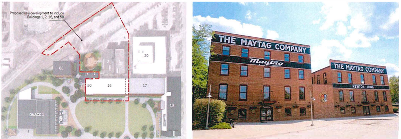
Figure 7 Maytag Complex - Buildings 1 & 2
