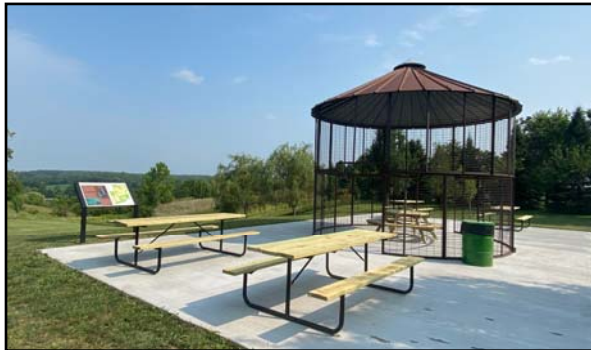
Above: The Calvin Winn memorial picnic shelter at Uhlenhopp Arboretum was made using an existing grain bin on the property.
