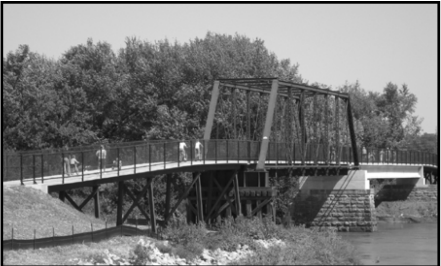
Main bridge on Union Bridge Trail in Woodbury County.
